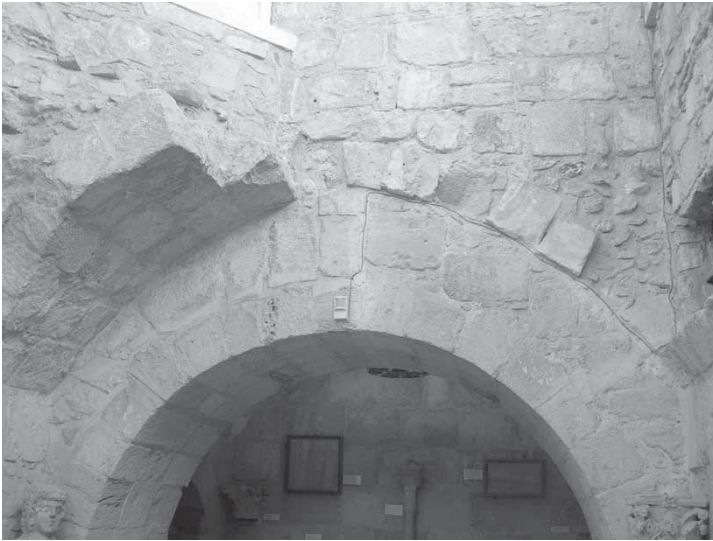
Fig. 39: Limassol Castle, upper level of cells, vestiges of barrel vault over the main hall [M. Olympios].
